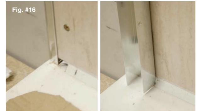
The panels can now be fitted on to the walls, positioning them onto the internal corner profile and resting on the Transeal bottom seal profile. The panels should be installed using 'Mermaid panel adhesive', which works in conjunction with the profile system to ensure a secure fixing.
