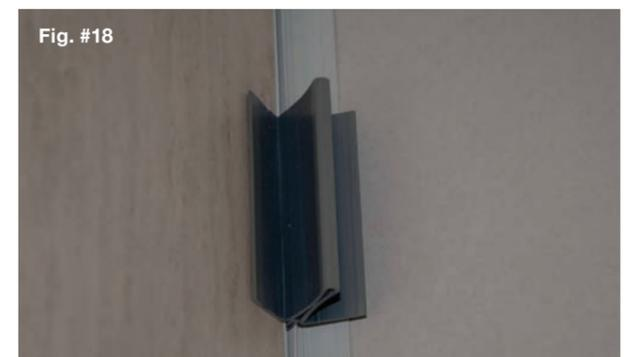
In conjunction with the hidden screws described in paragraph one the panels can be held temporarily in the corners using the corner brace tool (Fig #18).
