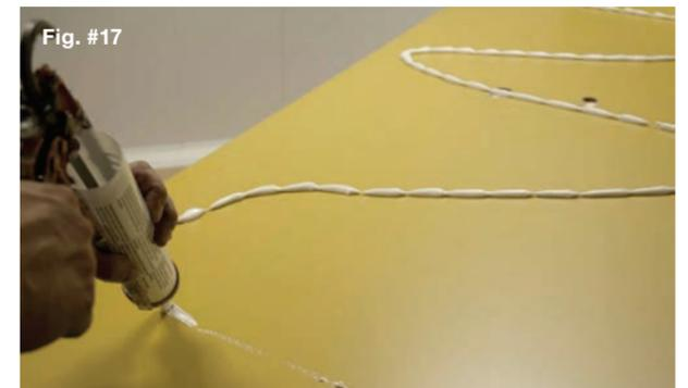
The adhesive has quick grab but long curing time. As the adhesive cures in air this may take a long time if ventilation to the glued areas is limited, it is imperative that mechanical fixings are therefore used in conjunction with the adhesive.
