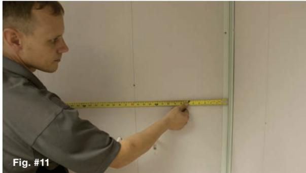
To determine the width of the panels, measure from the location pips (Fig #11). This should be checked at the top, middle and bottom to check that the walls are true. Panels may need cutting to suit where the walls are not square.
